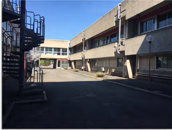
Figure 2: The “Sogene” complex. This structure comprises two main portions, and the one hosting the classrooms was ready since the end of 1986. The offices were essentially ready during the first half of 1988, and the Department settled in toward the end of 1988. When the Engineering and Economics Schools moved to their final destinations, the space allotted to the Physics Department nearly doubled.
